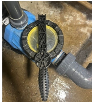
Close the pump filter using the handle provided
