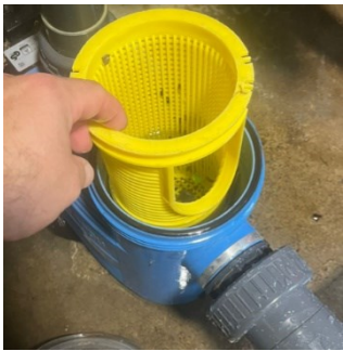
Once the filter is clean, then reinsert the filter
