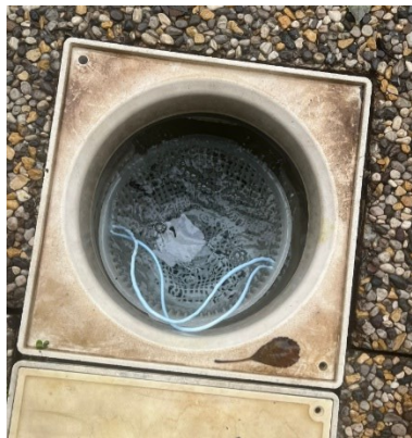
Insert the basket and chlorine basket in the hatch
