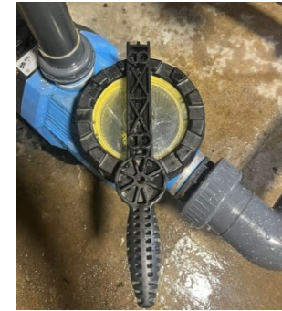
Open the pump filter using the handle provided
