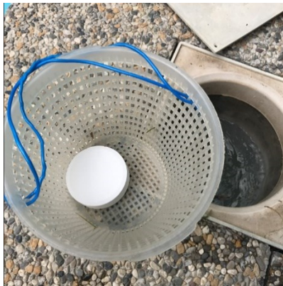
Clean the basket Add the chlorine tablet inside. (If you need chlorine 85, there are in local machine
