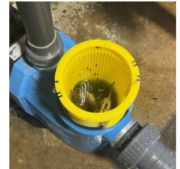
Remove the yellow filter, remove leaves and other debris
